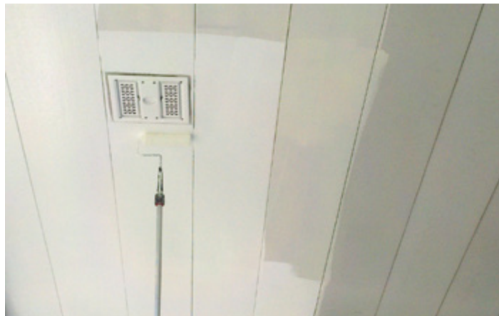
Shown: canopy painting in progress
