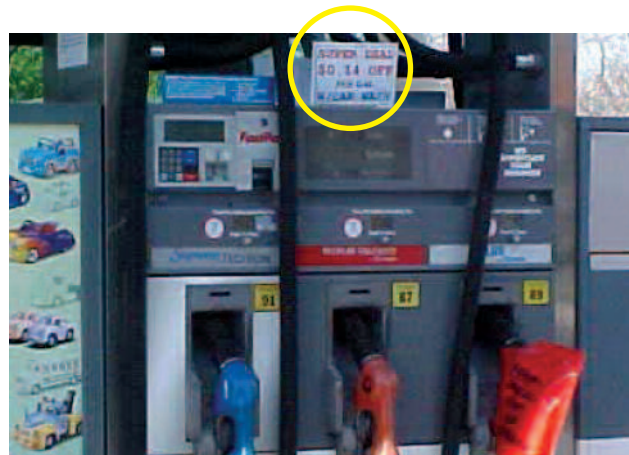
Replace with authorized pump topper signage.
