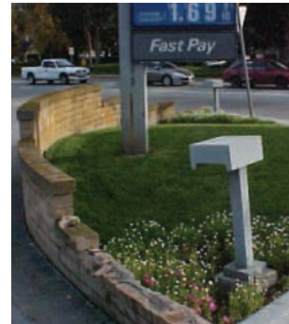
Repair damaged structures.
