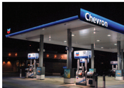
Canopy is in good condition; lights are operational and clean.
