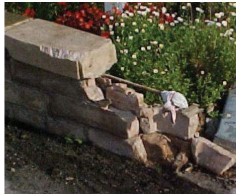
Repair damaged structures.
